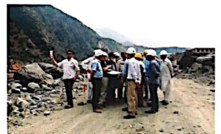
Work in Progress on KKH-01
